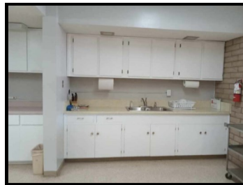
Remodeled kitchen—west side
